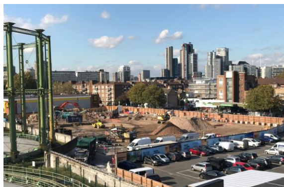
1 st Block Ground Prep
