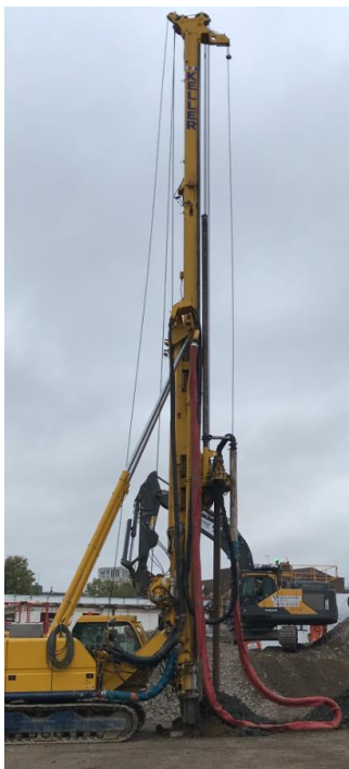
Piling Rig – From Mid-November
